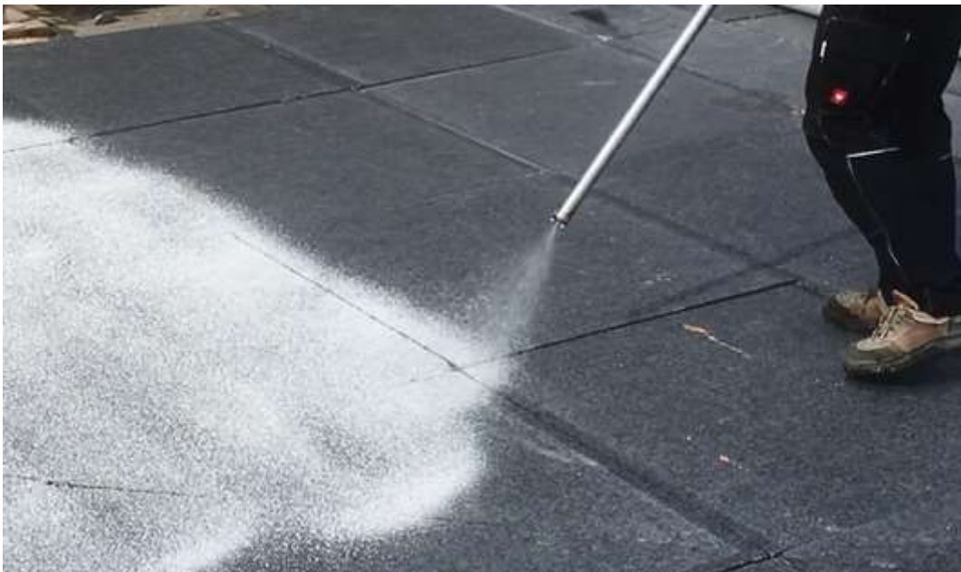
Application example: Full-surface adhesive application of a sprayable PU roofing membrane adhesive.
