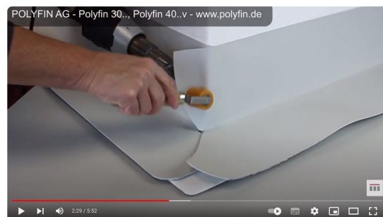
POLYFIN roof light corner with 1 patch Polyfin 1020
