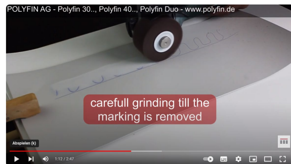
POLYFIN FPO TPO pre treatment weather exposed membranes
