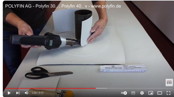
POLYFIN FPO/TPO - sealing of a pipe penetration
